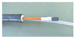
Remove insulating tape, and cut heater wires about 80 mm from end. Attach terminals as described in manual.
