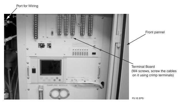
Figure 5.1 Wiring Work for Stack Gas Analyzing system
