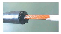
5. To discourage water or corrosive gas from entering the end of the piping bundle, paint end with sealant. It takes 24 hours for the sealant to dry completely, so after painting do not move it for 24 hours.
